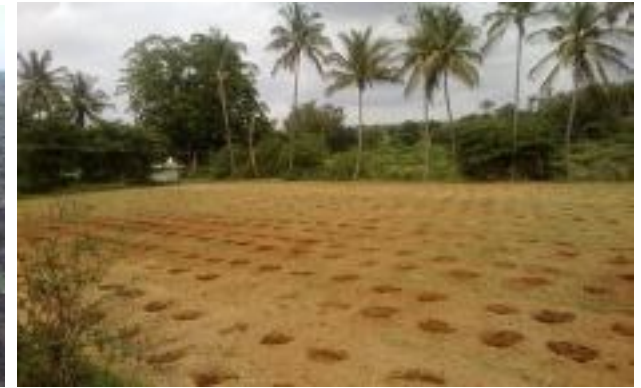
Marking and Pitting
