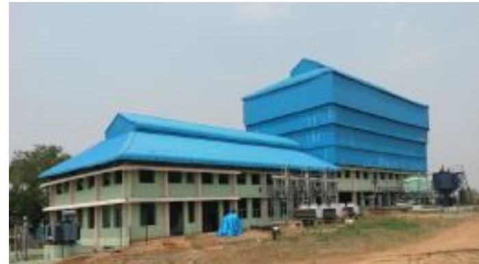
Power Plant, Gadag
