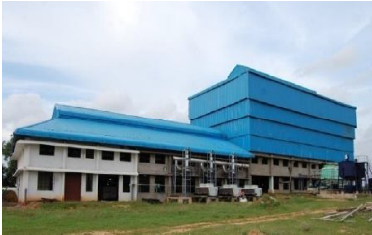
Mundargi Power Plant
